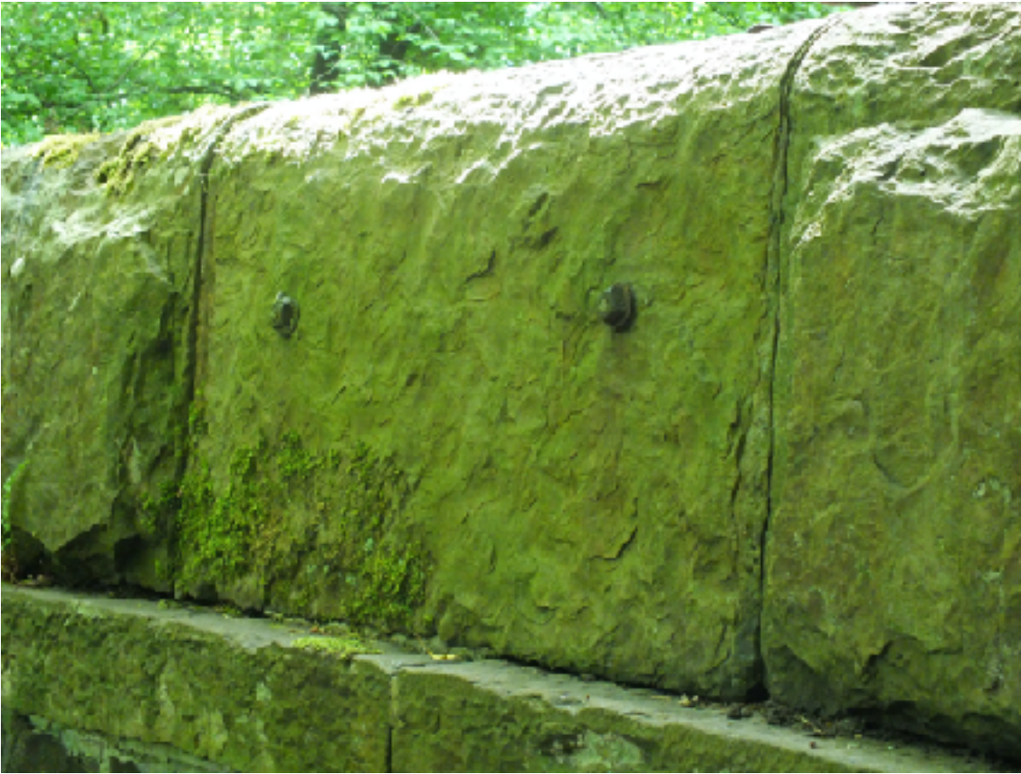
Image 7 Water side of the split parapet stone showing nuts on bolts
