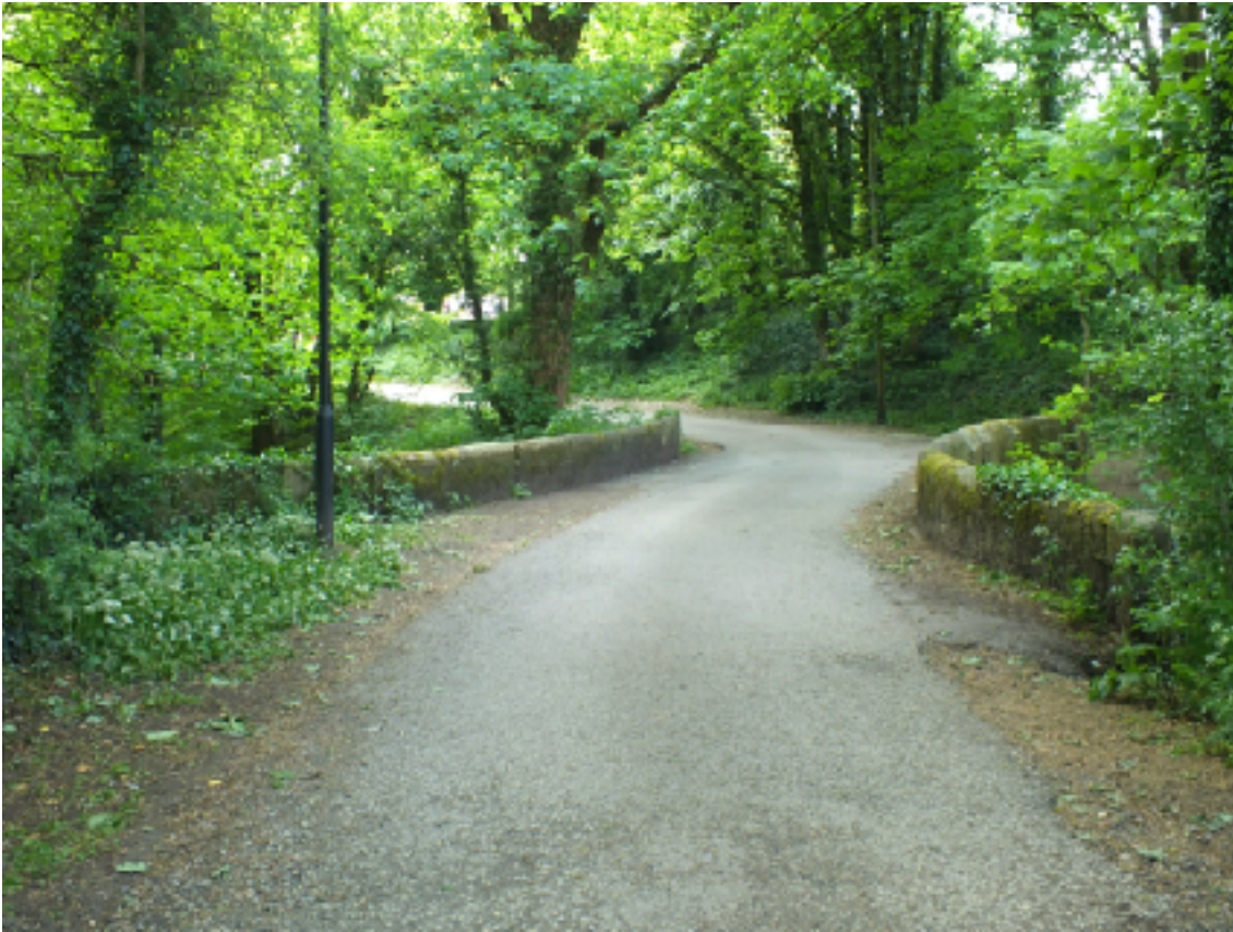
Image1, View of the Bridge on Hoggs lane, towards the A6
