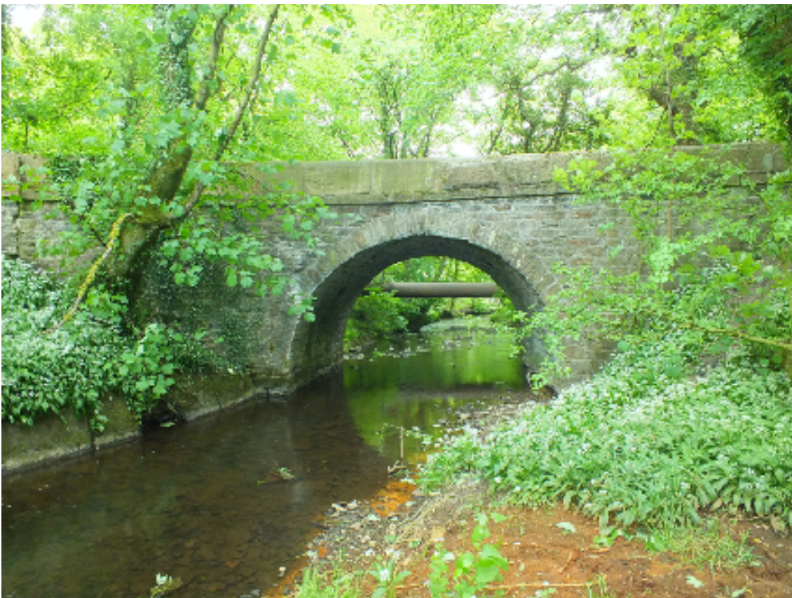
Image 2 View of the bridge, upstream side.
